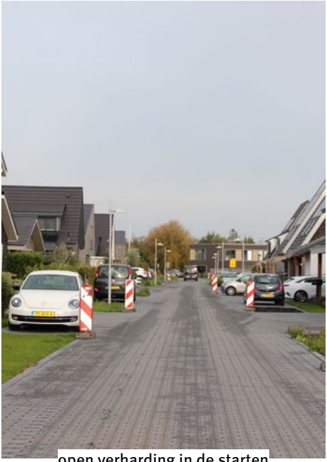
open verharding in de starten
