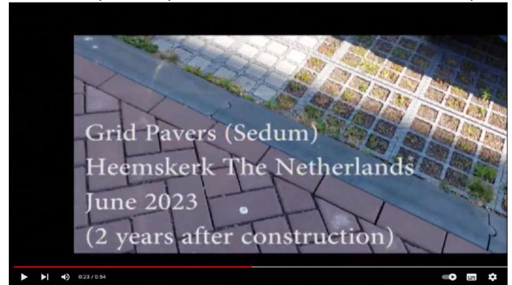
Grid Pavers permeable pavement sedum Heemskerk The Netherlands Testfield 2021 and 2023
